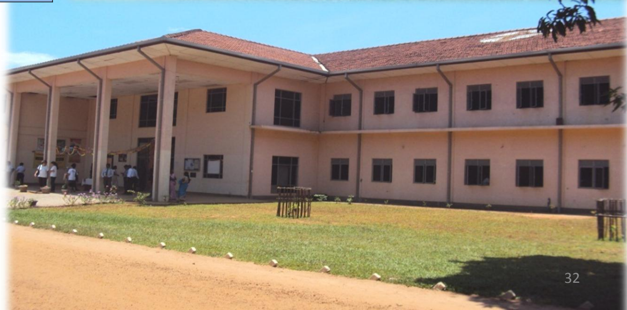
Refurbishment of Hospital Building District Government Hospital - Mullaitivu
