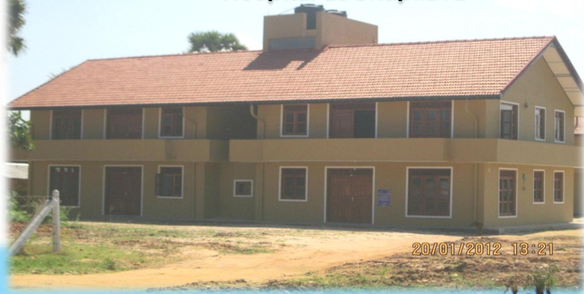
Re-construction of MO Qtrs. at District Hospital at Unapilavu
